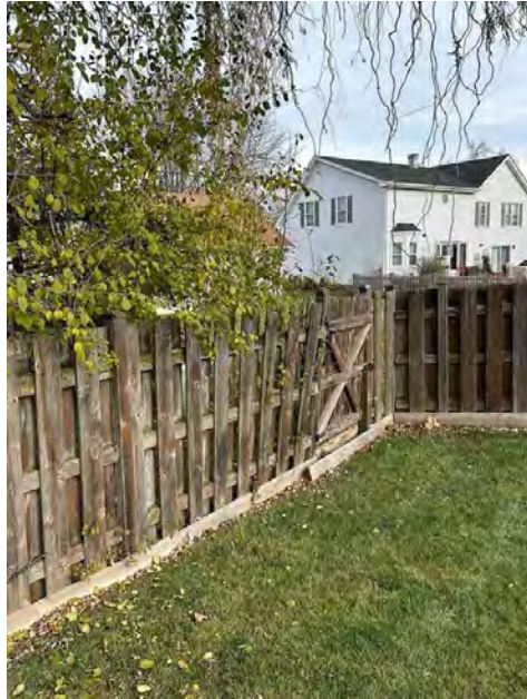
North Exterior- Repair
