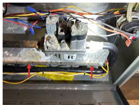
Have further evaluated and repaired/replaced
