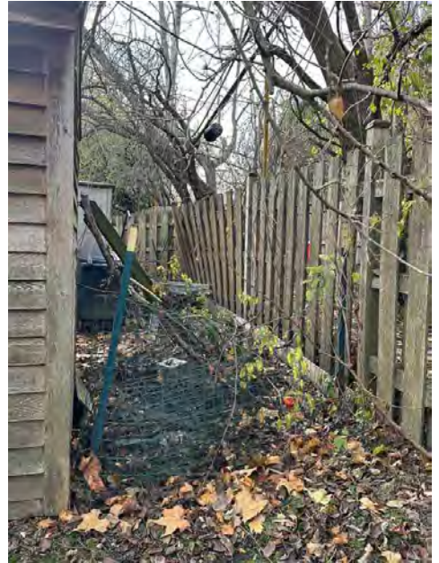
West Exterior- Repair
