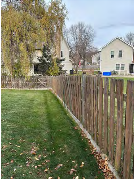
East Exterior- Repair
