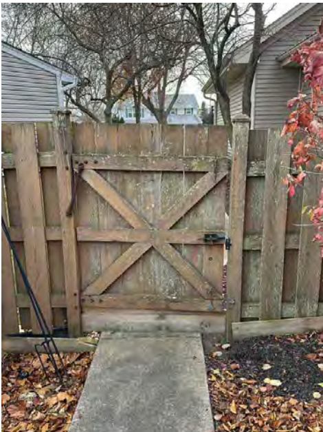
East Exterior- Repair
