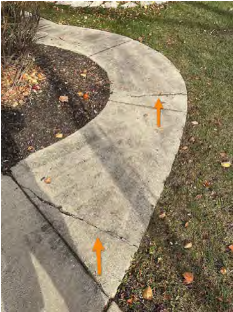
East Exterior- Repair
