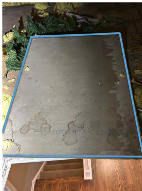
Suggest insulating and weather stripping
