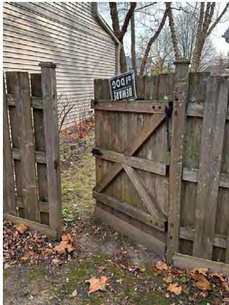
West Exterior- Repair
